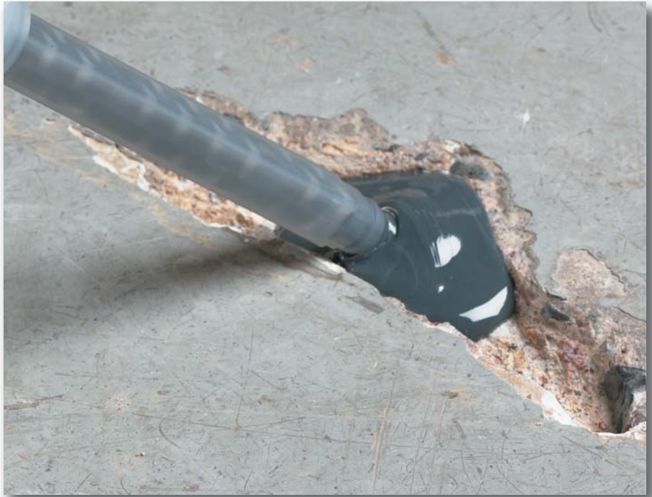
50ml and 12 fl. oz. duo-pak cartridges, 5-gallon pails, and 55 gallon drums are available to meet your production volume requirements. Nozzle automatically and precisely meters, mixes, and dispenses two-part urethane formulation. Apply material precisely where needed to conserve material. 157
