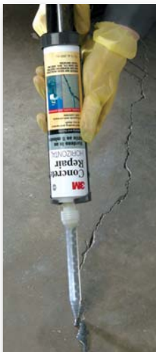
Self-leveling 3M™ Concrete Repair 600 flows smoothly into cleaned cracks and gaps and hardens in as little as 5 minutes. 156
