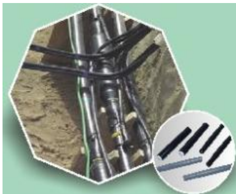
6. Cable Joints: For connecting two cable sections, and ensure that the extension of cable length.
